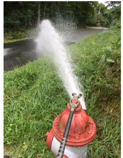
One of the things we do to keep water from becoming stale is to flush hydrants. This is also beneficial to our fire department as it exercises valves and provides a record of pressure and flow that can be expected from each hydrant.
